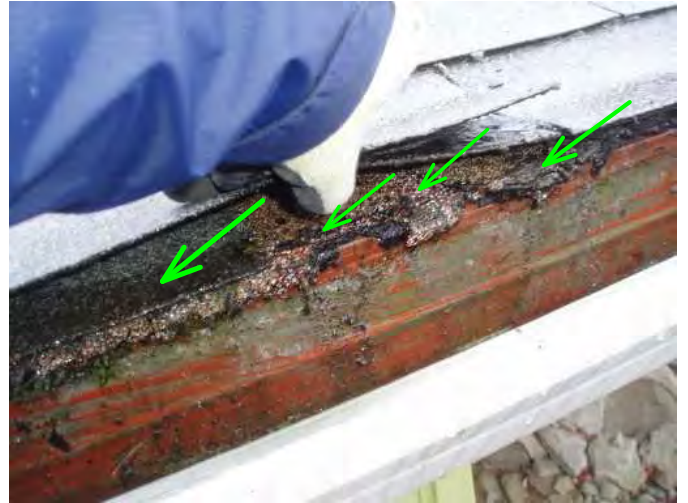
two layers of roof are noted...top layer is secured well...
