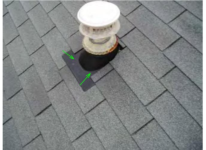
flashing are newer and plastic resin type...good...
