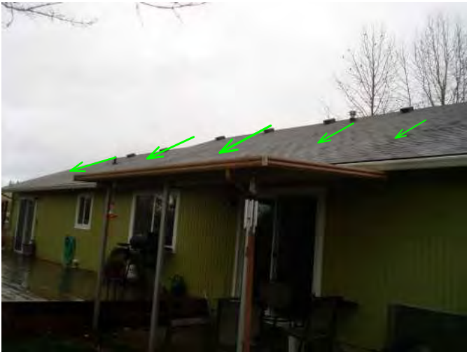
view of back roof is noted as draining fine...
