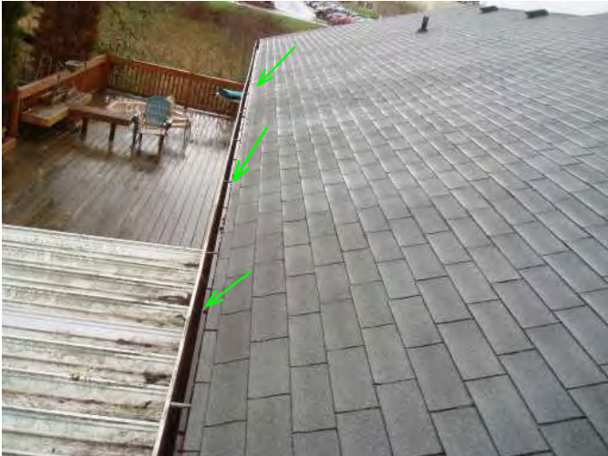
gutters are solid to home and draining well here as well...
