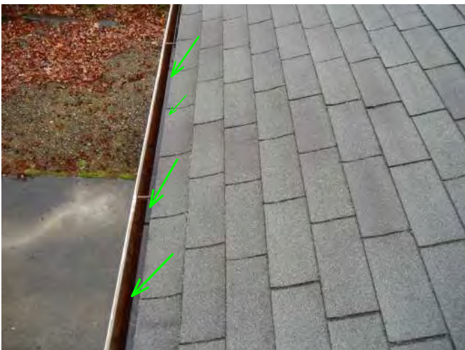
front of home has gutters operating well and draining and clean....good...
