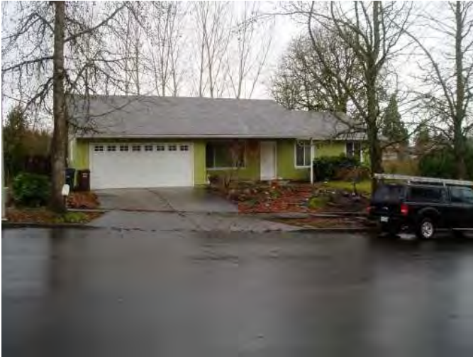
street view of home...all downspouts are draining into exits....fine...
